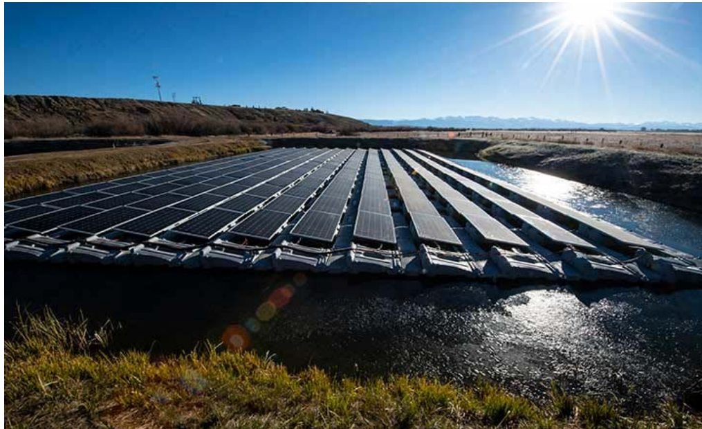
Floating PV array on a water retention pond. Photo by Dennis Schroeder, NREL
