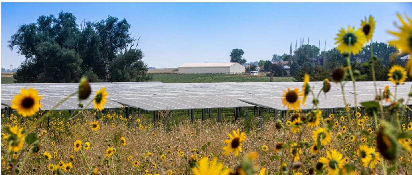
Photo by Werner Slocum, NREL 65601
