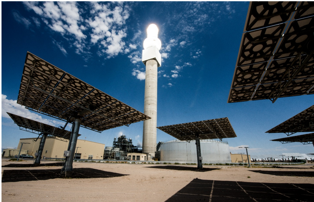
Figure 3. 110-MWe Crescent Dunes Solar Energy Project in Tonopah, Nevada, with 10 hours of thermal storage
