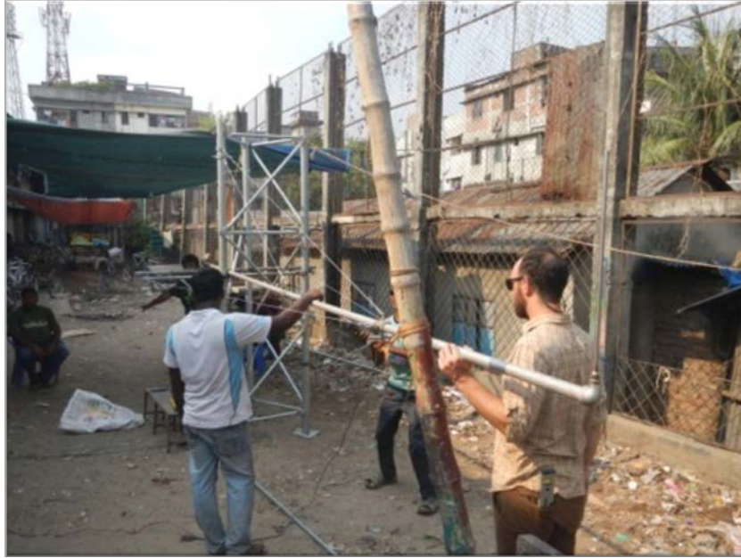
Figure 15. Mounting boom testing. Photo by Harness Energy.
