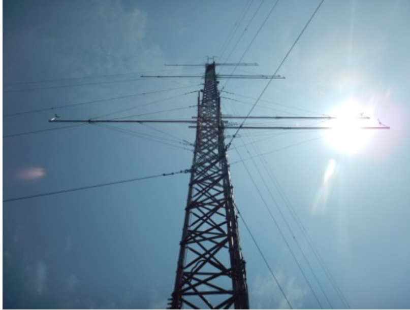
Figure 12. Typical MET tower configuration with sensors attached to boom extensions. Photo by Harness Energy.
