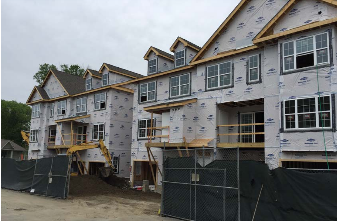
Figure 1. Avalon Green III under construction
