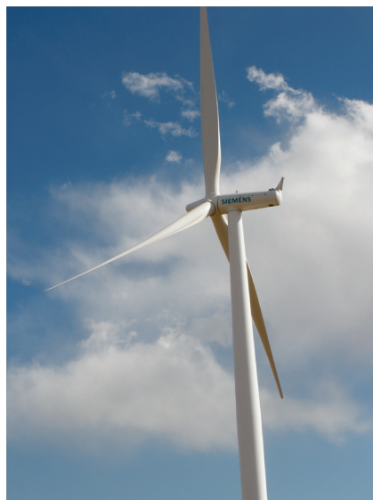
The Siemens 2.3 MW turbine is among the largest land-based turbines deployed. Its rotor diameter is a whopping 331 feet – more than the length of a football field.
