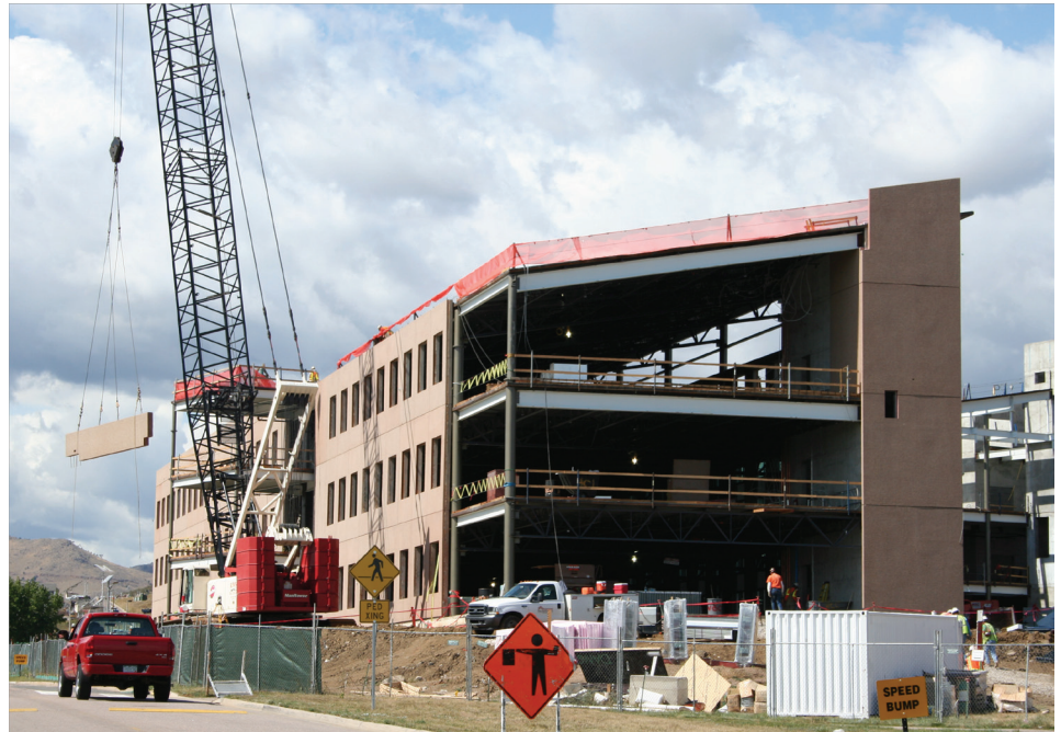
The exterior panels on the Research Support Facilities benefit the building on many levels. The exterior keeps the weather out and helps regulate interior temperatures. The middle section provides insulation and the opposite side serves as the interior wall.
