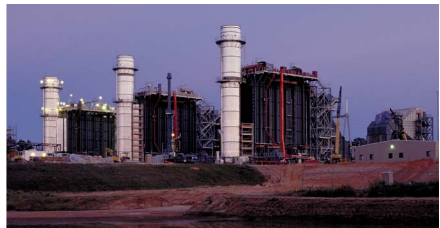
Combined Cycle Power Projects
