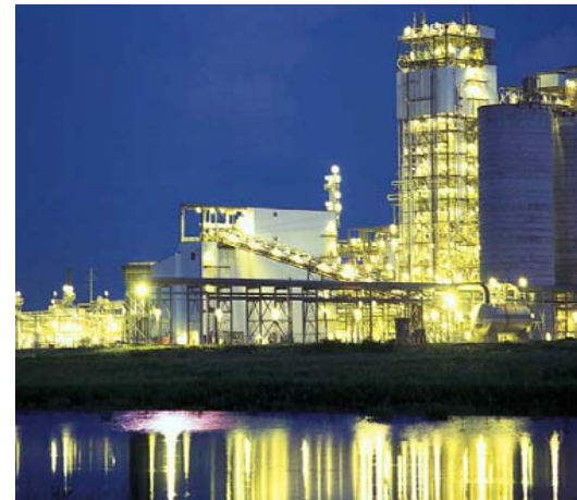
Polk IGCC Power Station
