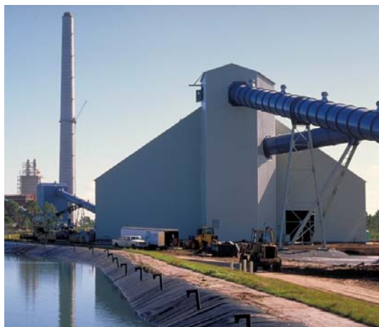
Indiantown Cogeneration Station
