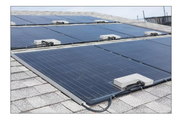
**Glass-less modules attached** using an adhesive approach
