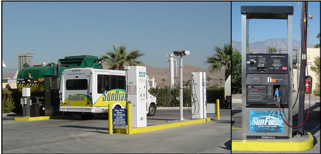
Figure D-1. Public fueling at SunLine's Thousand Palms CNG fueling station (left) and a CNG dispenser (right)
