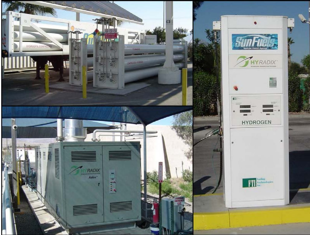
Figure D-4. SunLine's hydrogen storage (top left), HyRadix Adéo commercial reformer (bottom left), and hydrogen dispenser (right)
