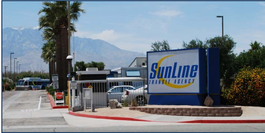
Figure B-2. SunLine headquarters in Thousand Palms
