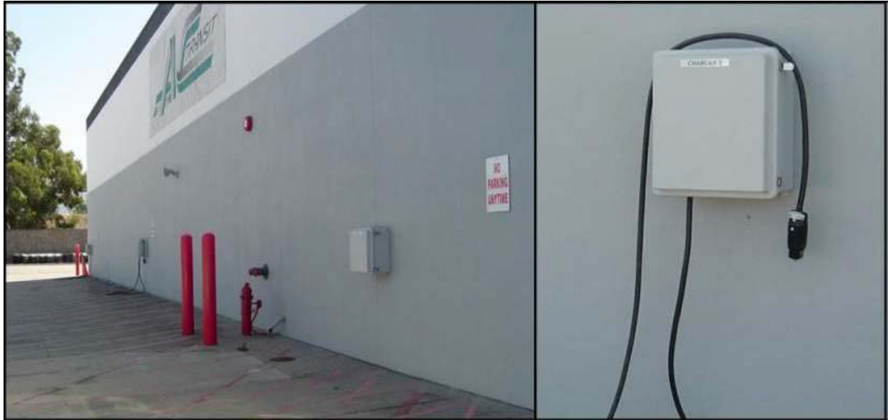
Figure D-4. Fuel cell bus/battery charging station at AC Transit (Photo credit: L. Eudy, NREL)
