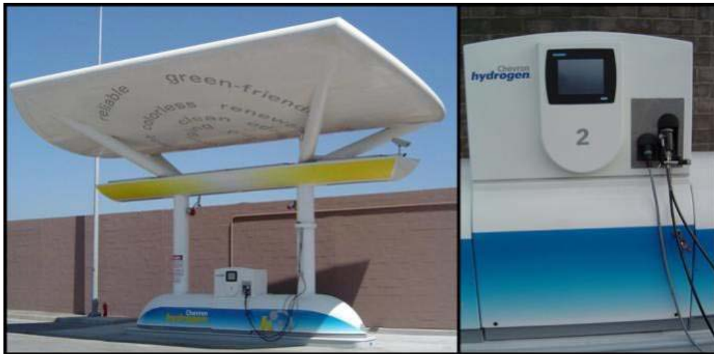
Figure D-1. Dispenser at Chevron—AC Transit Energy Station (Photo credit: L. Eudy, NREL)
