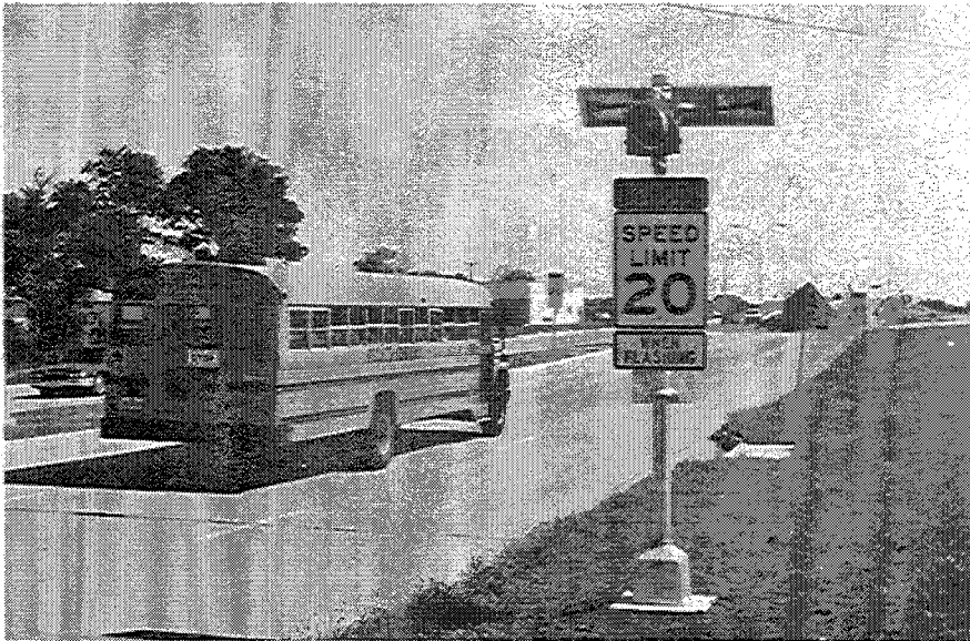
Figure 8 Photovoltaic traffic signal
