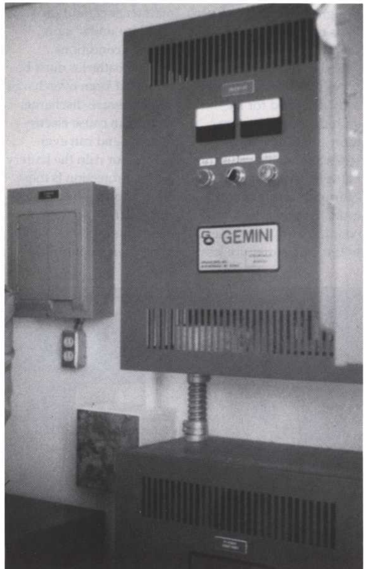
Power conditioners are used in many systems to maximize power output, change the dc electricity from the PV array to ac electricity, match the converted ac electricity to a utility's ac electrical network, and to protect the utility network system and its personnel from harm during repairs.
