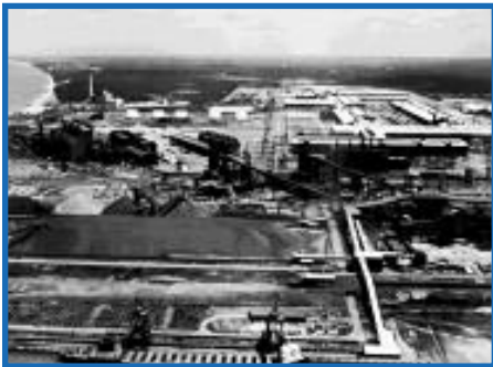
Aerial view of the Burns Harbor Division, Bethlehem Steel Corporation
