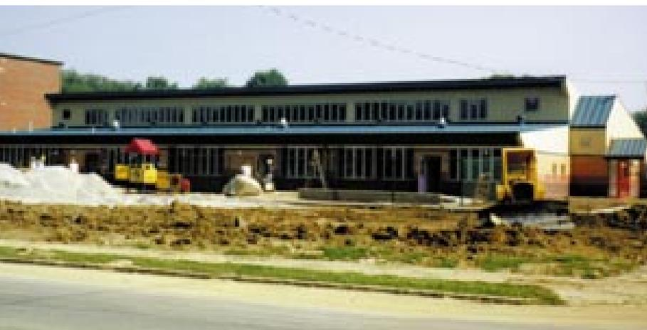
**The 10,550 sq.ft. design for the St. Benedict Child Care Center in Louisville, Kentucky, takes advantage of the sun's heat and light with its atrium and its large, south facing and clerestory windows. The air core flooring system captures and stores energy from solar and internal gains, creating a radiant heating effect. Overhangs avoid unwanted solar gain during summer months.**
