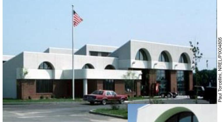
**The Emergency Services Building in Valmeyer, Illinois, uses whole-building design to reduce mechanical system and electric lighting requirements. By incorporating daylighting, direct gain and natural ventilation systems, and high-efficiency HVAC equipment, lights, and energy management system, the building is expected to use 60% less energy and save over \$8000 per year.**
