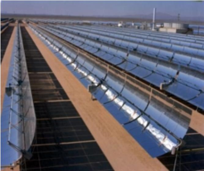
**Figure 1 SEGS V Parabolic Trough Solar Thermal Power Plant [KJC Operating Company]**
