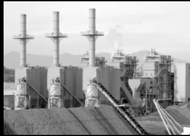
This 50-MW biomass power plant located in Anderson, California, runs on residues produced by nearby companies in the forest products industry.
