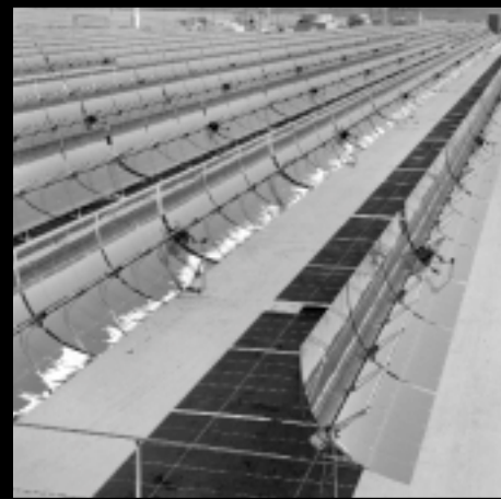
This solar power plant located in the Mojave Desert in Kramer Junction, California, is one of nine such plants built in the 1980's. During operation, oil in the receiver tubes collects the concentrated solar energy as heat and is pumped to a power block located at the power plant for generating electricity.
