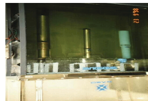
33. Shenzhen - Sinosolar PV Pumps Demo
