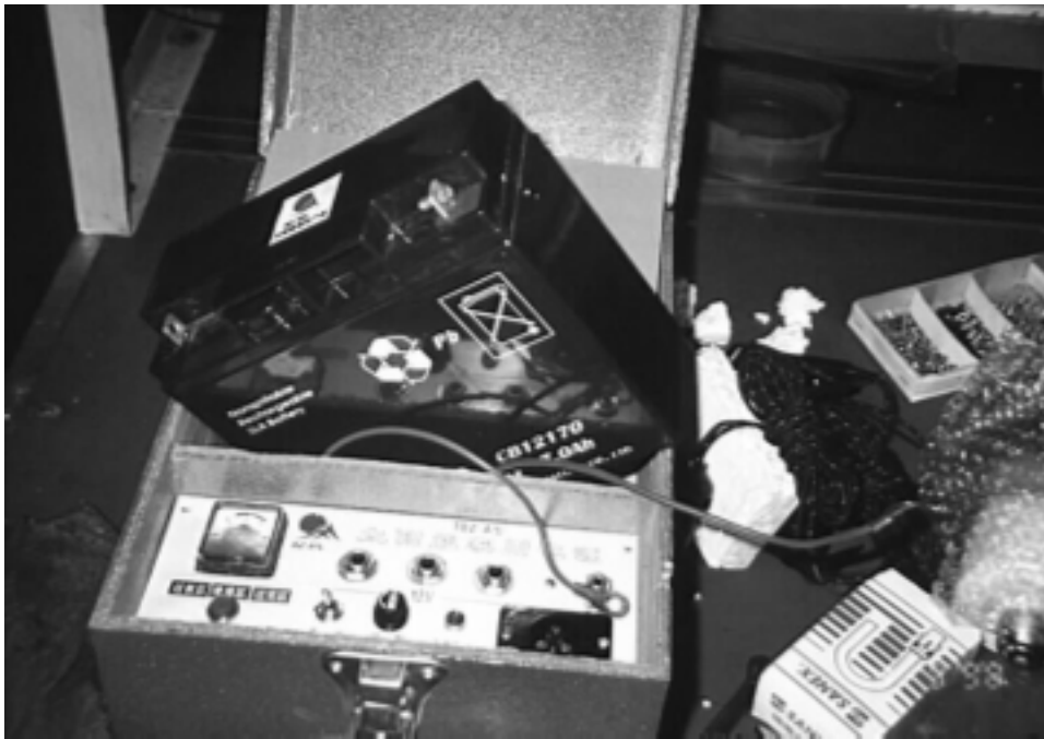
Figure 1. Typical solar home system
