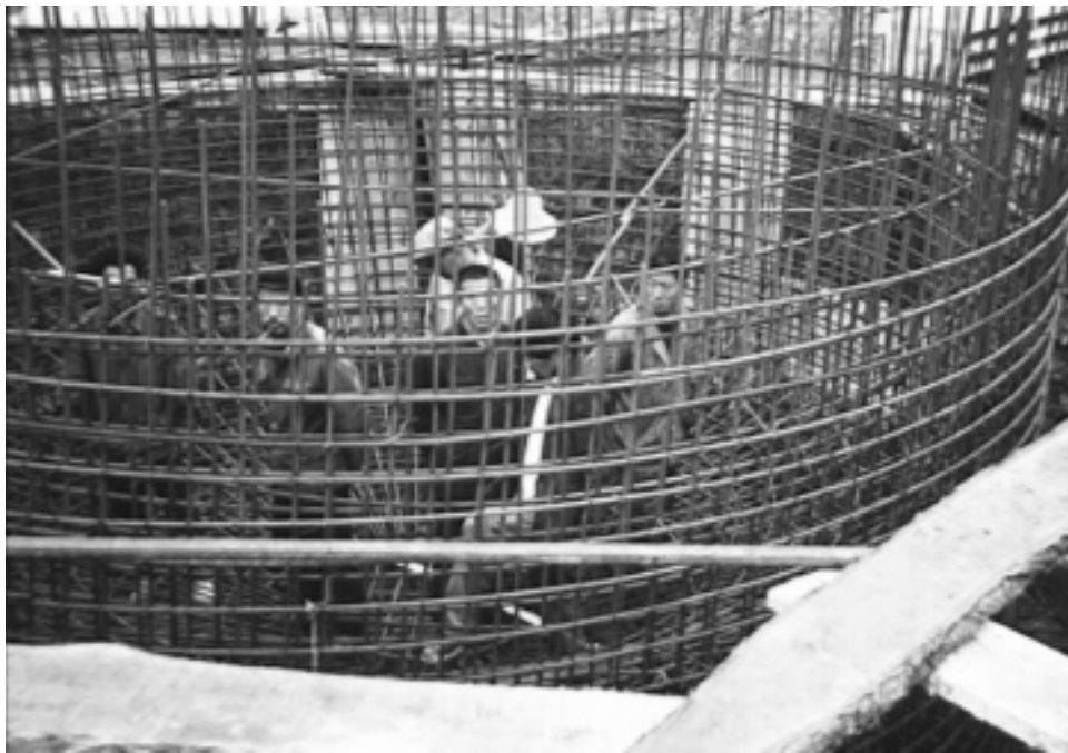
Figure 8. Collection tank under construction for biomass system
