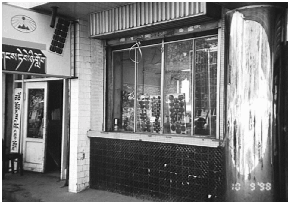
Figure 3. Typical solar shop
