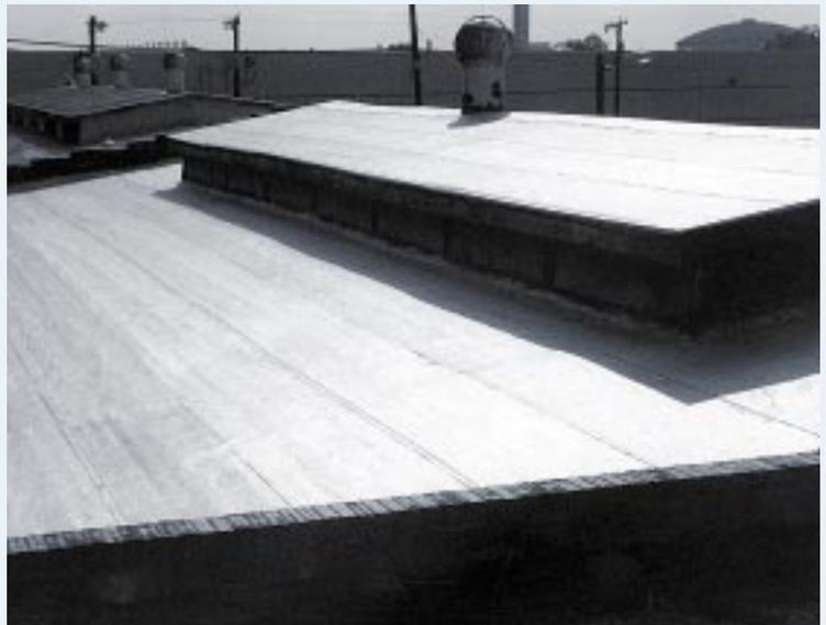
**Aluminum chips form a highly reflective surface on asphalt roofs, cutting down on heat absorption by the dark pigmented asphalt, and decreasing the need for air conditioning inside.**
