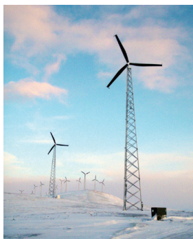
Photo by Dennis Schroeder, NREL 16307
