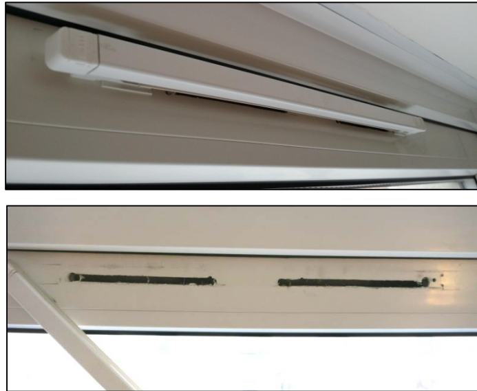
Figure 28. Typical trickle vent in open position (top) and with cover removed (bottom)
