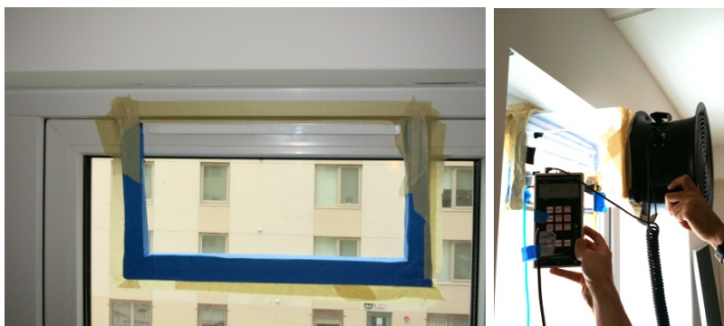
Figure 29. Setup for testing airflow through trickle vents
