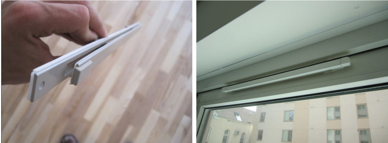
Figure 9. Common trickle vent (left) and installation in a window frame (right)
