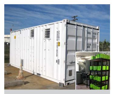
The energy management system installed at the Pacific Missile Range Facility holds the system's main controller, advanced batteries (shown in the inset) with power conditioning equipment, and the human machine interface.
