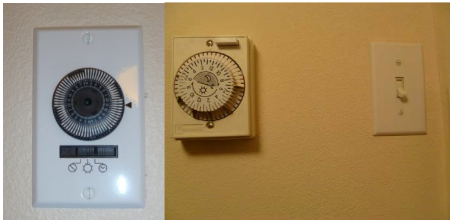
Figure 3. Exhaust ventilation system controls
