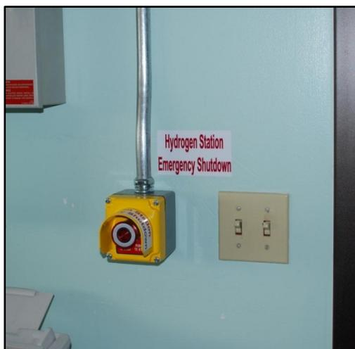
**Figure 12. An emergency stop control was added to the Emeryville Division Control Center**
