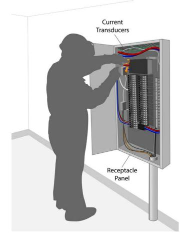
Figure 2 This study required that metering be installed to capture PPL energy use intensity. Illustration by Al Hicks
