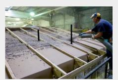
Improved attic insulation strategy relying on dense-packed or compressed batt insulation in shallow attic area near the roof eaves. Area-weighted average insulation value of R-45 is achieved.
