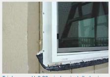
Triple-pane U-0.20 window installed using improved pan flashing and air sealing practices, compared to current factory processes.
