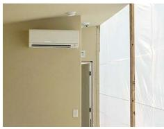
Views of factory-installed ductless mini-split heat pump system that eliminates the need for ductwork in the home and arrives on site complete and ready to operate.
