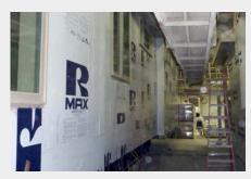
Rigid foam sheathing reduces thermal bridging in conventional R-21 2×6 framed wall assemblies. .75-in. polyisocyanurate sheets yield R-5.
