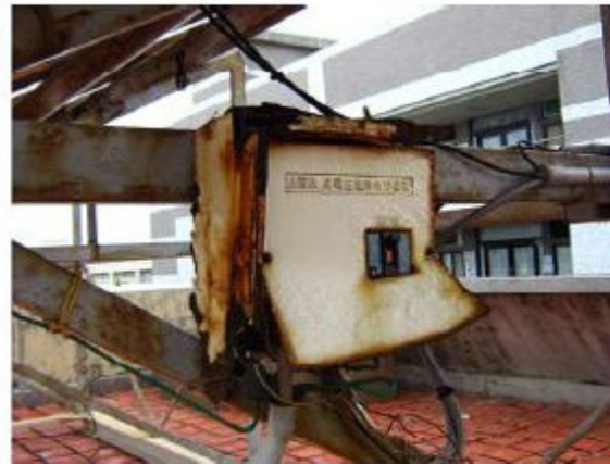
Corrosion in a harsh environment
