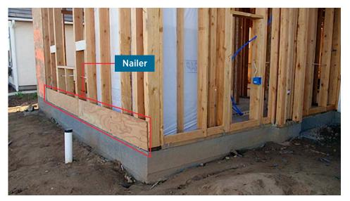
The slab edge of the test house prior to installation of the XPS rigid foam insulation, showing the nailer that supports the foam.
