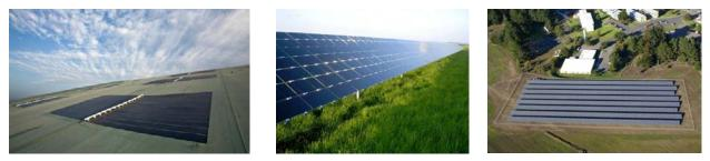
Figure 4. Thin-film solar panels installed on (left) solar energy cover and (middle and right) fixed-tilt mounting system. *Pictures from (left) Republic Services, Inc., 23817; (middle) Beck Energy, NREL 14726; and (right) U.S. Coast Guard Petaluma site, NREL 17395*
