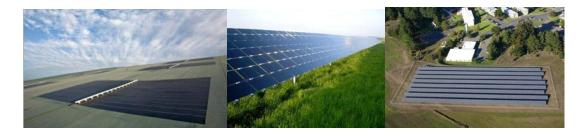
Figure 4. Thin-film solar panels installed on a (left) solar energy cover and (middle/right) fixed-tilt mounting system. Photos by (left) Republic Services, NREL 23817, (middle) Beck Energy, NREL 14726, and (right) U.S. Coast Guard Petaluma Site, NREL 17395
