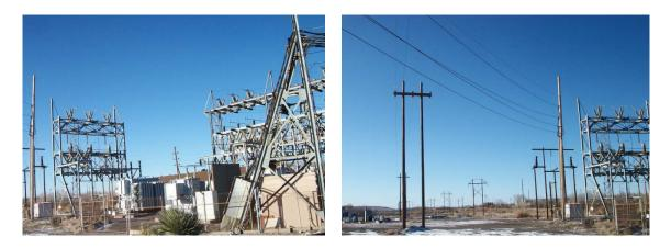
Figure 10. Electrical tie-in point of 24-kV and 115-kV lines for the PV system at the Chino Mine. Photos by Kosol Kiatreungwattana and Lars Lisell, NREL
