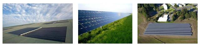
Figure 4. Thin-film solar panels installed on (left) solar energy cover and (middle/right) fixed-tilt mounting system. *Photos from (left) Republic Services, NREL 23817, (middle) Beck Energy, NREL 14726, and (right) U.S. Coast Guard Petaluma Site, NREL 17395*
