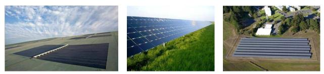
Figure 5. Thin-film solar panels installed on (left) solar energy cover and (middle/right) fixed-tilt mounting system. *Photos by (left) Republic Services Inc., NREL 23817, (middle) Beck Energy, NREL 14726, and (right) U.S. Coast Guard Petaluma Site, NREL 17395*
