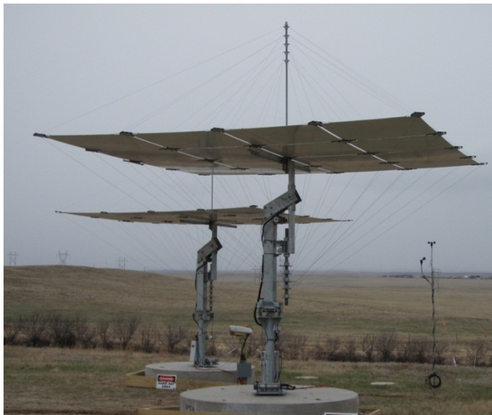
Figure 1 Two Solaflect Energy Baseline Heliostats in Stow Mode 60% to 65% Less Steel per Square Meter at Baseline
