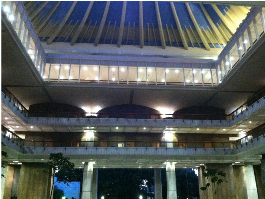
Figure 16. Nighttime exterior metal halide lighting at Hawaii State Capitol building Photo by Ian Metzger, NREL
