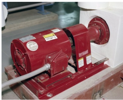
Figure 7. Example of premium efficiency pump motor
