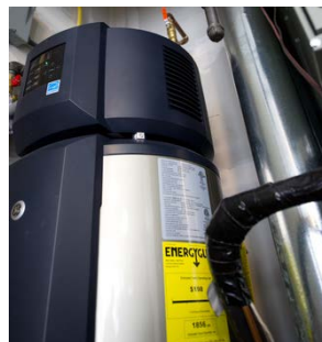
Figure 8. Example of heat pump service water heater
