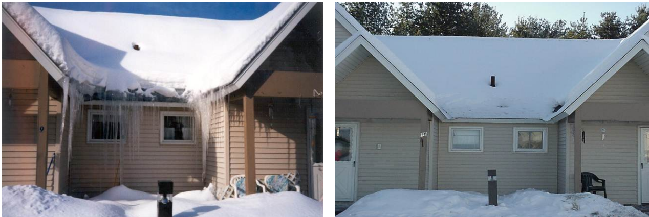
Figure 2. Before (left) and after (right) air sealing penetrations into any unconditioned roof cavities (Housing Vermont 2010) (Photos courtesy Efficiency Vermont)
