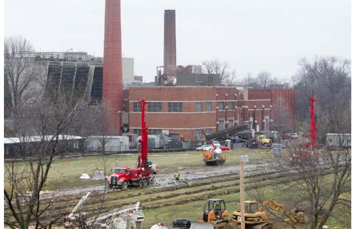
EERE sponsored Ball State University’s campus-wide geothermal system, which is expected to save \$2 million annually in operating costs and cut the university’s carbon footprint in half. Here, geothermal boreholes are dug to install the system next to an existing coal-fired power plant. *Photo from Ball State*
