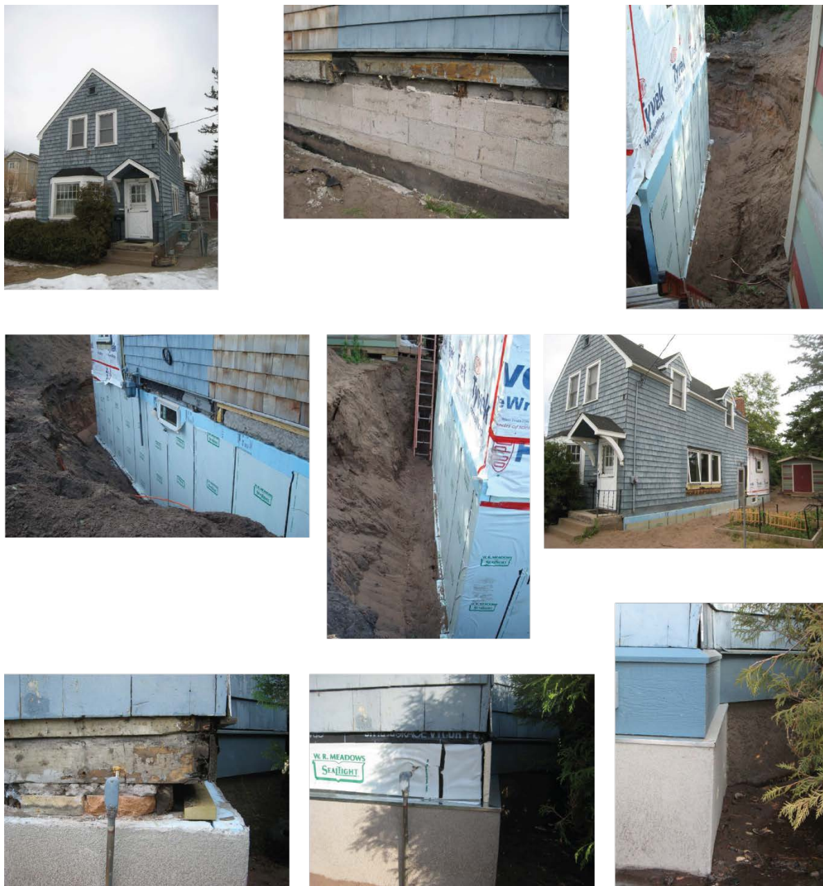
Figure 6. Full foundation excavation and insulation in Duluth
