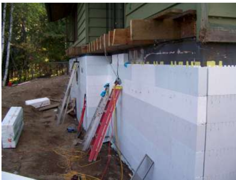
Figure 5. Installation of 4-in. EPS R-ETRO
