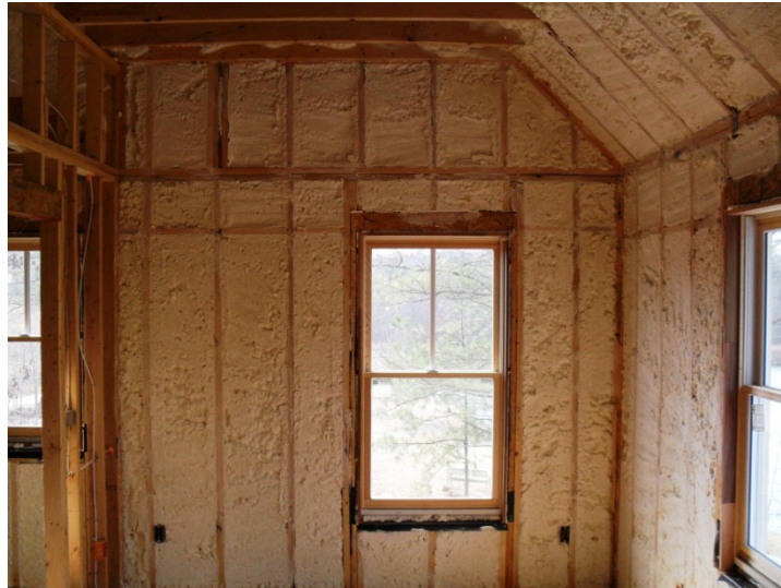
Figure 5. Insulation at second floor and roof, Nest Cottage nine
