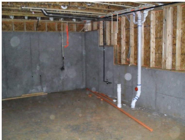
Figure 3. Foundation wall and framing, Nest Cottage nine
