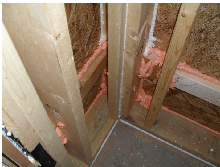
Figure 4. Air sealing detail at exterior basement wall corner, Nest Cottage nine
