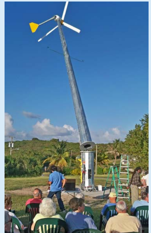
The tower of the wind turbine installed at the St. Croix Reformed Church and Kingshill School can be hydraulically raised or lowered depending on weather conditions. Photo from Don Buchanan, VI Energy Office, NREL/PIX 20816
