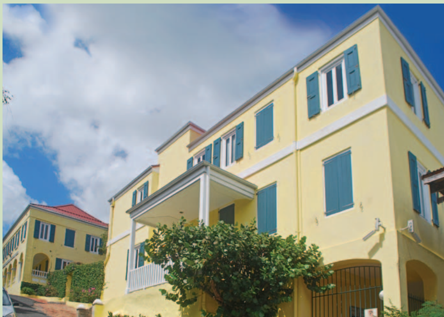
The Bjerget House received major energy efficiency upgrades through the Southeast Energy Efficiency Alliance (SEEA) Worthwhile Investments Save Energy (WISE) program. Part of the U.S. Department of Energy's (DOE's) Better Buildings Program, WISE works with local governments to educate citizens about energy efficiency building upgrades in their communities. EDIN-USVI clean energy workshop attendees will have an opportunity to tour the Bjerget House and see energy saving upgrades firsthand. Photo from Quality Electric Supply Inc., NREL/PIX 20812
