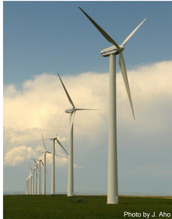
Fig. 1. A row of turbines in a wind plant located in Alberta, CA. This wind plant contains 114 horizontal axis wind turbines (HAWTs), each rated at 660 kW with a rotor diameter of 47m and hub height approx. 50m.
