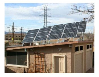
Fig. 5. Photograph shows shadows of power lines that are cast across the panels in the late afternoon.
