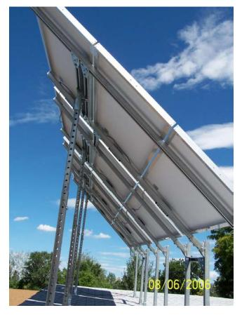
Fig. 4. Photograph of the back row of panels on the detached garage showing the  $40^\circ$  tilt.
