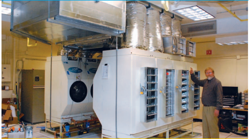
The above photo shows the multi-stage indirect evaporative cooling units installed at the National Snow and Ice Data center in May 2011. Photo used with permission from the National Snow and Ice Data Center.
