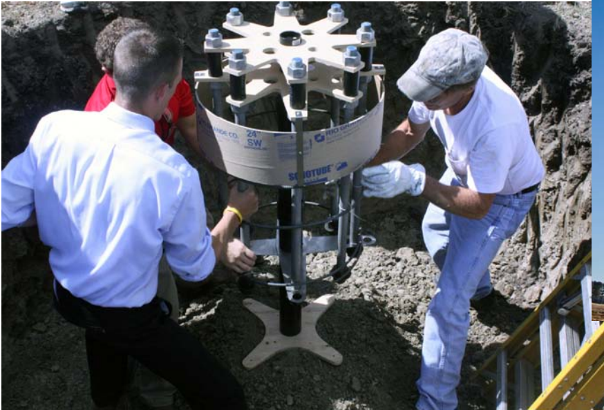
A team sets the SMART Foundation in place before the concrete pour for the Wind for Schools project installation at Eudora High School in Eudora, Kansas. Photo from Kansas State University, NREL/PIX 19692
