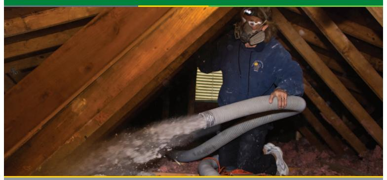
A weatherization crew member blows dense pack insulation into the attic and wall cavities of a client's home. *Photo from Simonson Management Services*
