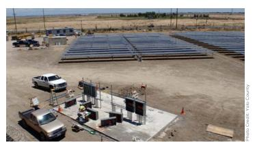
Figure 1. Installing the 1 MW ground-mounted solar PV system in Yolo County.
