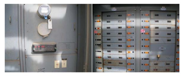
a) SCE main meter 3-029-1238-11 in main distribution & metering panel "MDP" at existing treatment plant located in center of plant.
