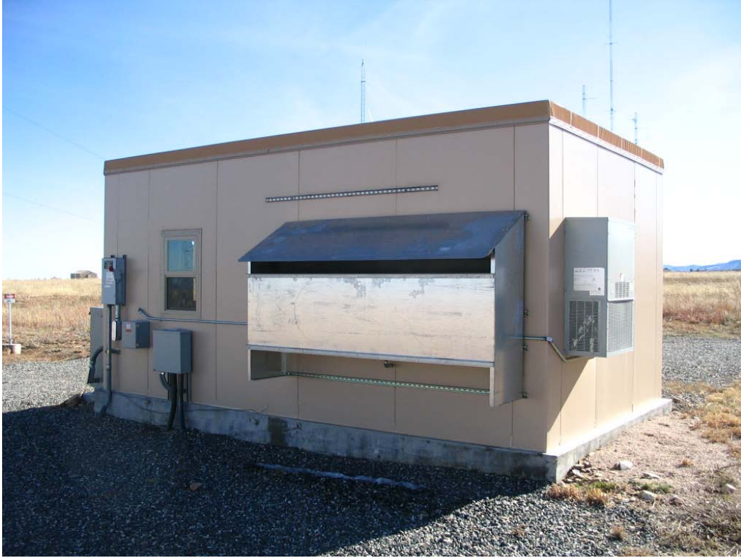
Figure 5. Diversion loads on exterior of data shed
