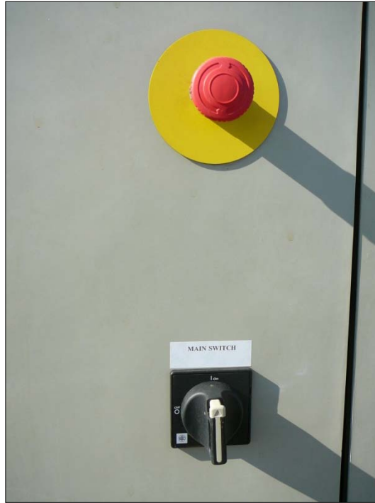
Figure 15. Gaia-Wind 11 kW emergency-stop button and main switch
