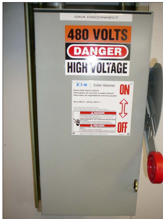
Figure 14. Gaia-Wind 11 kW disconnect switch
