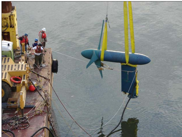
Figure 1. The Verdant Power 35-kW hydrokinetic turbine
