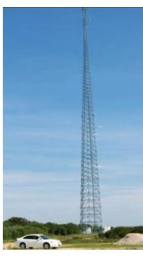
As part of a wind resource assessment effort with the U.S. Coast Guard, NREL provided Cape May (in New Jersey) with anemometers and wind vanes installed at 30, 44, 74 and 97 meters on an existing 109-m tower. Credit: Richard Ker, PIX 15661.
