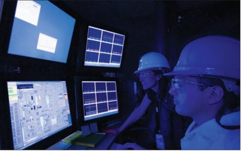
The Thermochemical Users Facility (TCUF) is equipped with sophisticated data monitoring and operation control systems. This control room simultaneously monitors all key operating parameters.
